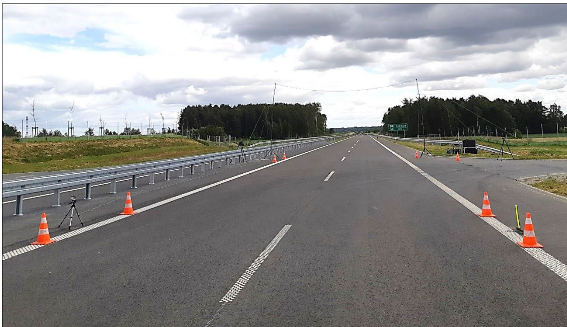
Figure 4. Measurement location at Szemud (Poland)
