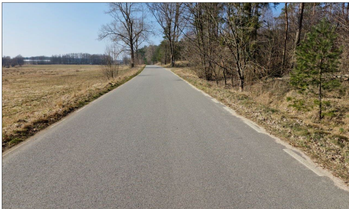
Figure 2. Measurement location at Bartoszylas (Poland)
